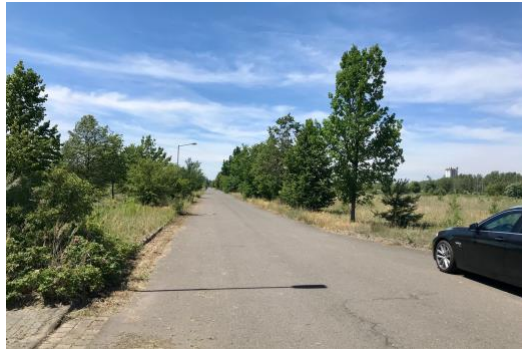
Internal roadway accessing AIG's industrial site
