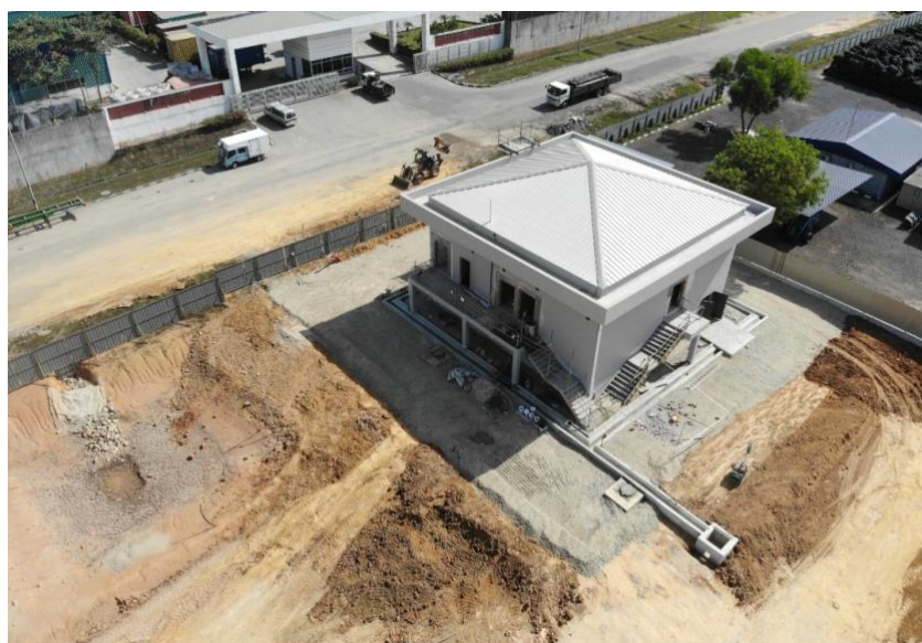
Figure 1 – Electrical substation construction progress March 2020 (South West aspect)
