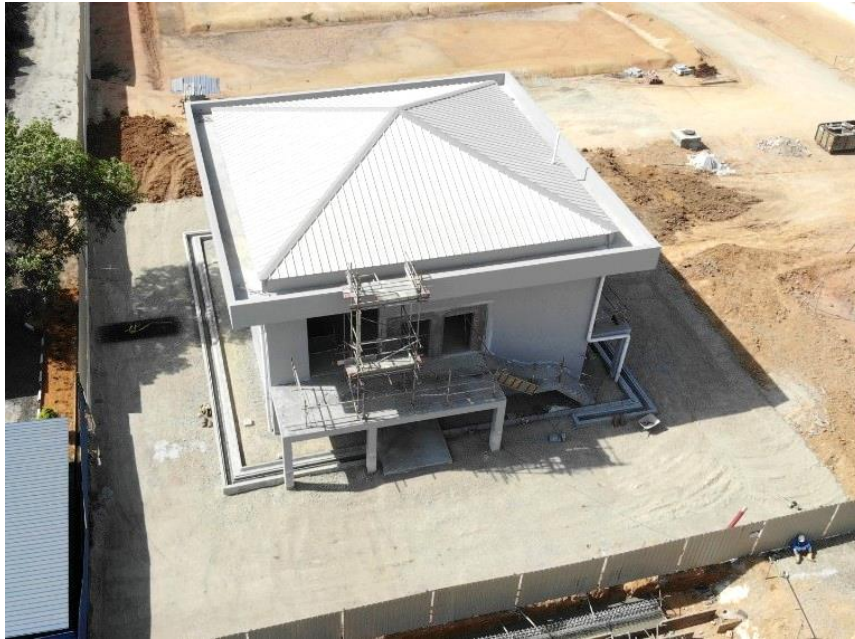
Figure 2 – Electrical substation construction progress March 2020 (North aspect)
