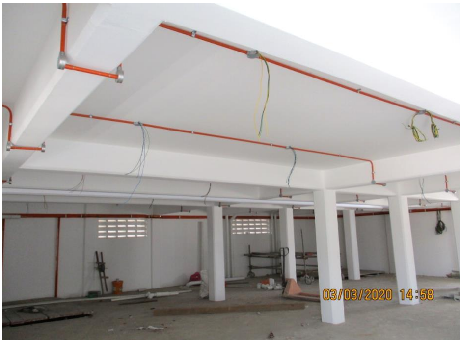
Figure 5 – Electrical substation internal detailing March 2020
