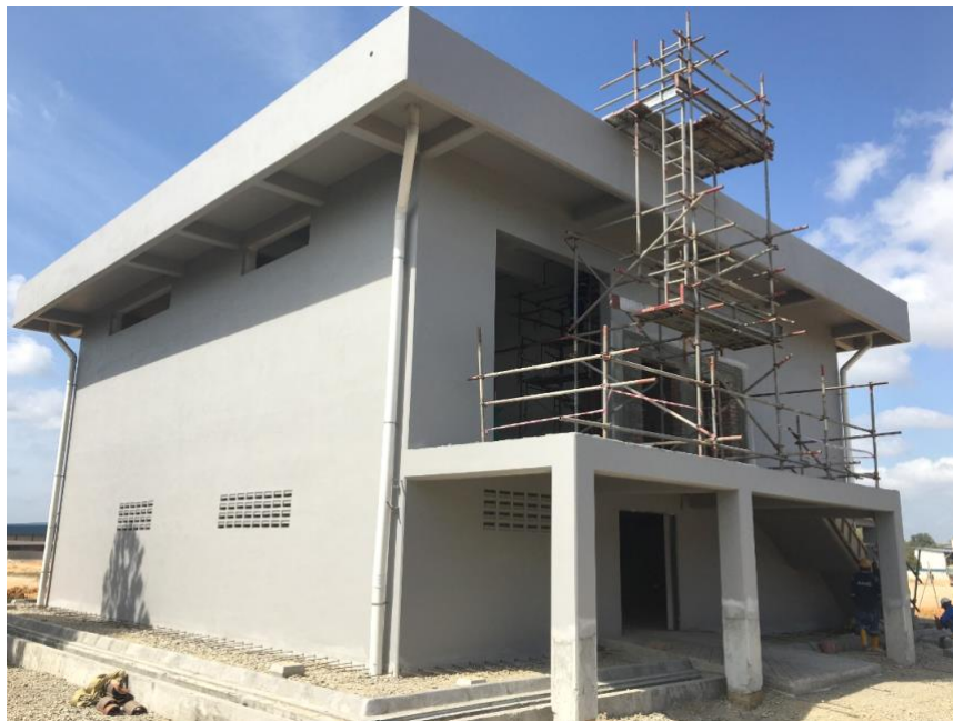
Figure 3 - Electrical substation construction progress March 2020
