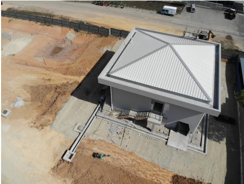
Figure 4 – Electrical substation roof completion March 2020
